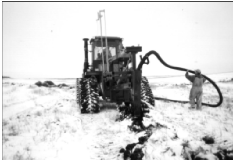
Installation of the tiling pipe in saline areas
